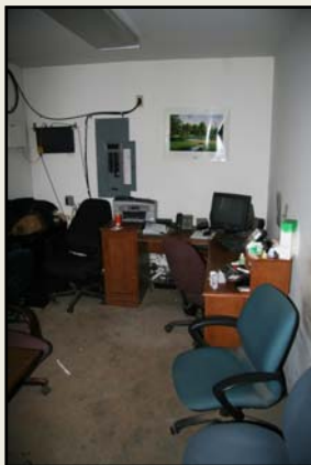
Office Area with Little Damage
