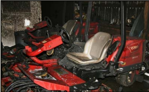
Mower Plastic Damage
